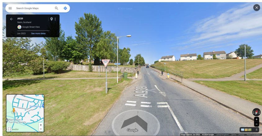
Existing pedestrian and National Cycle Route 1 crossing, looking North
